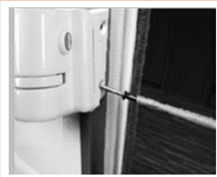
Insert 4 screws into the pre drilled holes.
