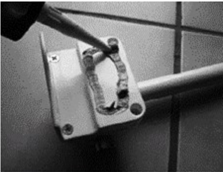
Apply sealant to frame.
