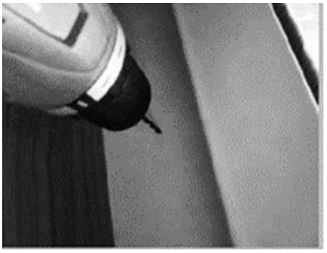
Check position of frame and drill centrally, screw frame in two places for extra support.
